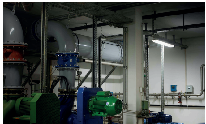
Safety under the most demanding conditions: From now on, the digital clamp-on ultrasonic flowmeter ensures high accuracy flow measurement of the return activated sludge – avoiding any complex installation
